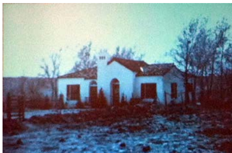
Photo of the house taken most likely in the 1940s.
